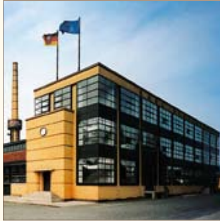
Fagus Factory, constructed by Walter Gropius in 1911
